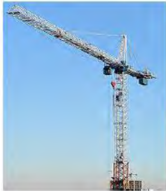
Gb. Tower Crane
