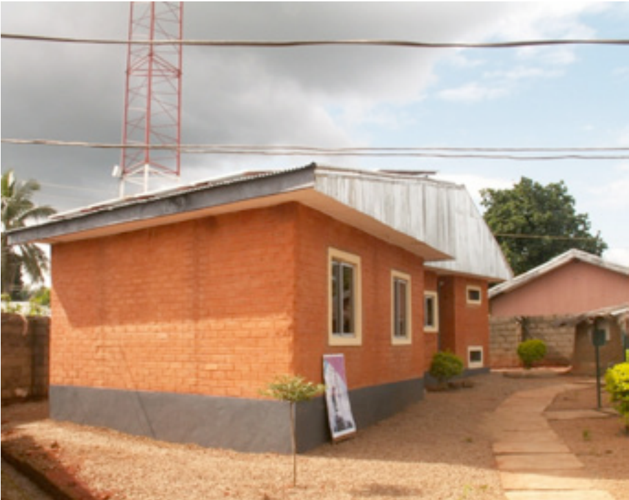
Figure 11.2: The NOC is built by locally made laterite brick stones, produced and laid by youths in Kafanchan.
